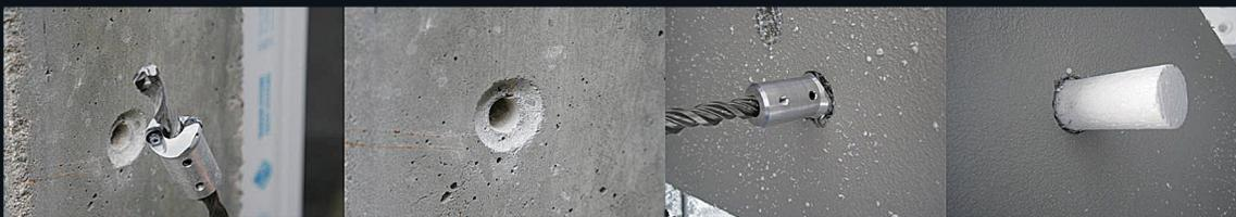
**ANKER MIT MONTIERTER SCHUTZHÜLSE, ZUM SCHUTZ BEI GERÜSTDEMONTAGE DER WÄRMEDÄMMUNG.**
